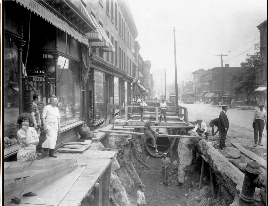
Williamsburg Conduit Construction | Source: DEP
