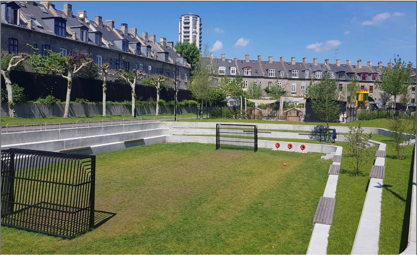
Water square in Carlsberg City, Copenhagen, Denmark. During extrememe rainfall events, the square can detain water to reduce the stress on the sewer system and prevent flooding in the surrounding areas. On dry days, the area provides space for recreation, athletics, liesure, and socialization. Source: Ramboll Group
