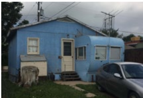
ABOVE: One of the houses within the Ponderosa Mobile Home Park community
