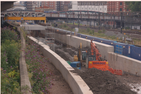
Figure 12: Crossrail Tunnel Royal Oak Portal Construction (Marcus Rowland, 2011)
