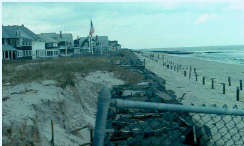
Figure 16: Exhumed portion of small rock seawall under dunes in northern section of Bay Head, New Jersey after a severe storm. Many residents were unaware that this seawall existed because it was completely covered by extensive dunes (Photograph by Dr. Susan D. Halsey).
