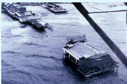
Figure 11: Damage to Atlantic City's Steel Pier from the March, 1962 storm. Note missing center portion removed by wave uplift during the height of the storm (Photo courtesy of Dr. Susan D. Halsey). 22
