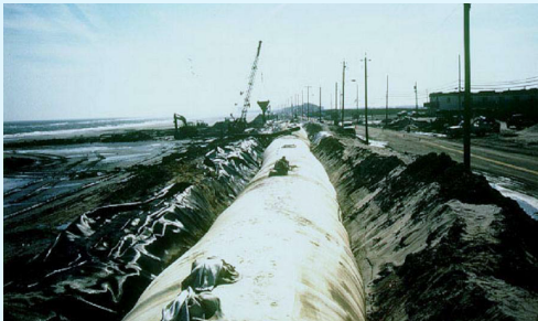
Figure 17: Sand filled geotube used to create the core of a protective dune line (Photograph by Dr. Michael S. Bruno).
