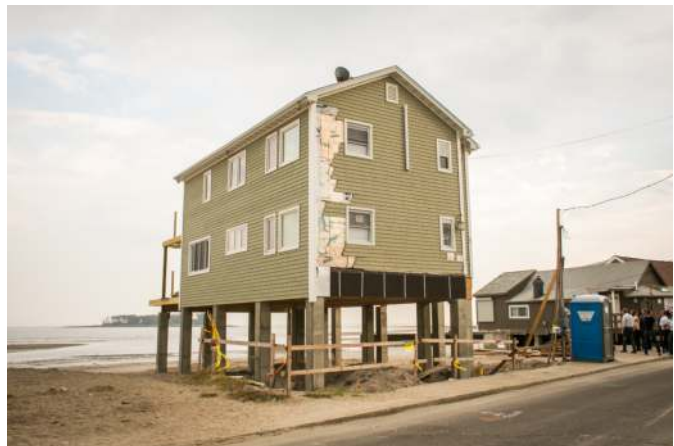
Cameron Baylock A waterfront home in Milford Connecticut is rebuilt to new ABFE standards.
