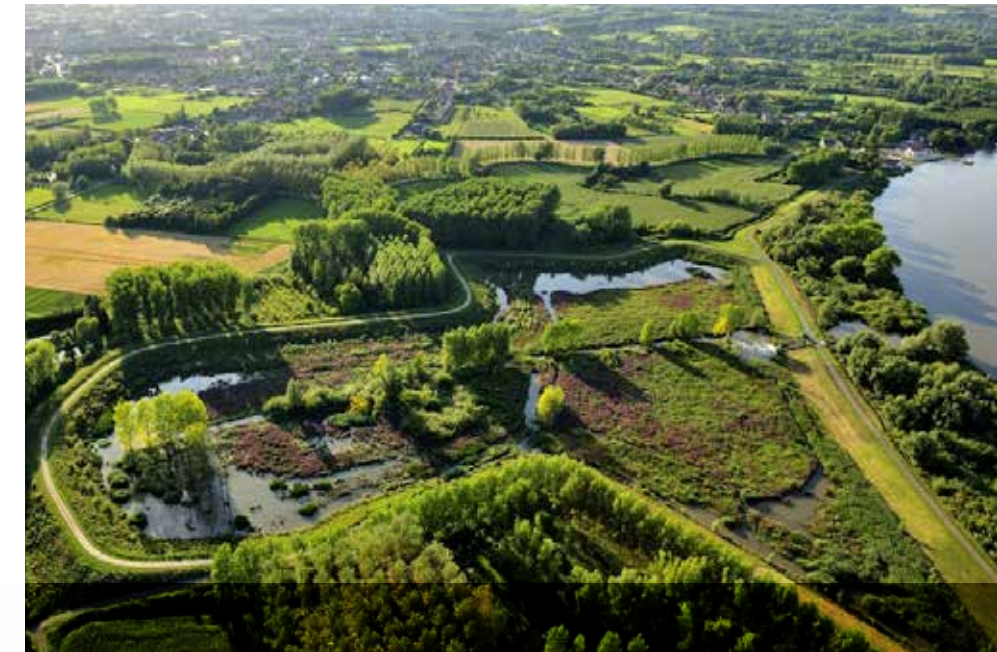
Westerschelde: example of a flood protection berm (right) and an outer berm (left)
